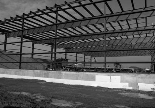
Miller Waste Compost Facility
