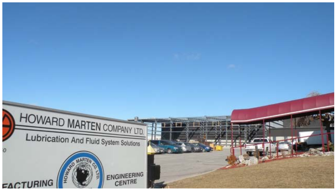
(Above) Howard Marten now putting finishing touches on new addition
