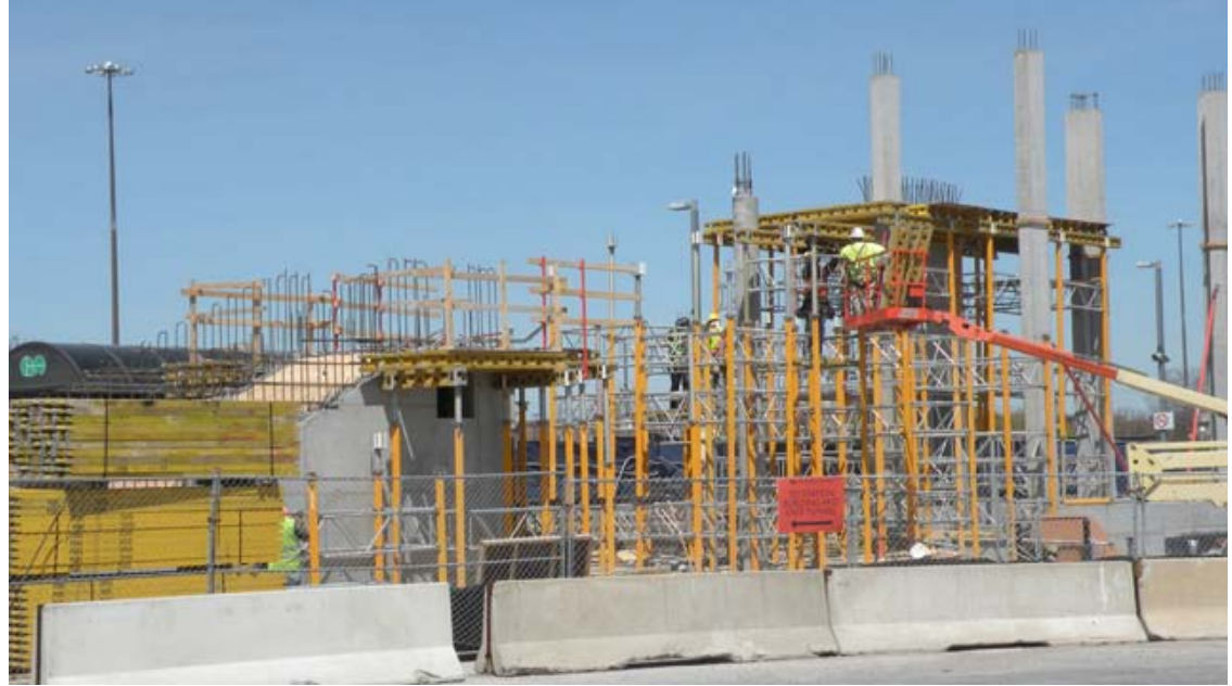
(Above) Construction of landing on south side of pedestrian bridge
