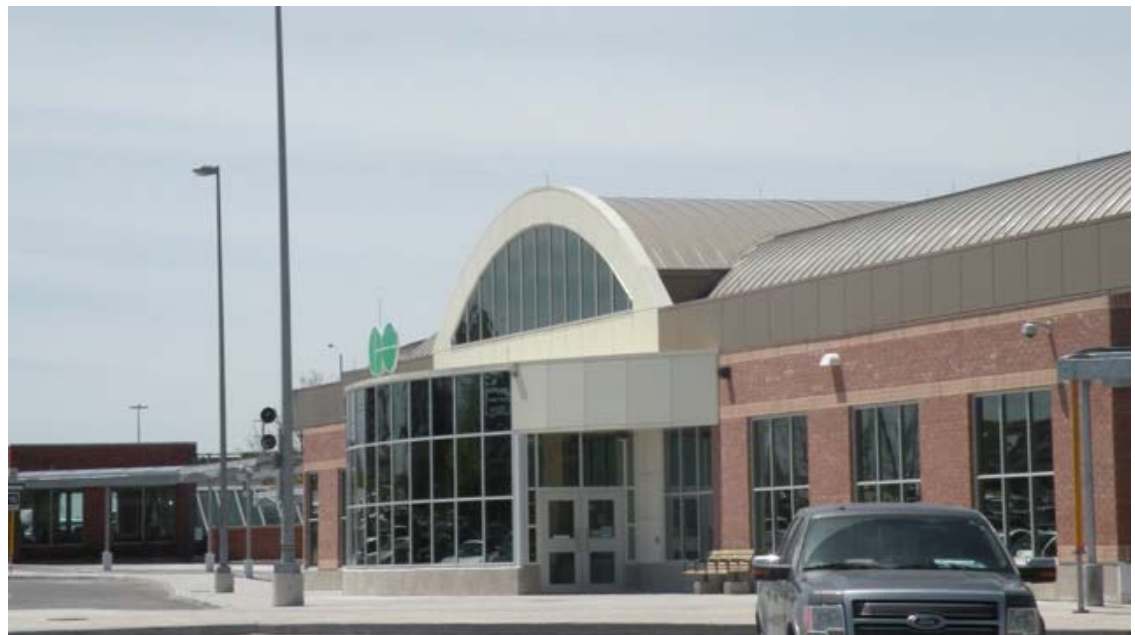
(Above) First LEED certified GO Transit Terminal in Ontario
