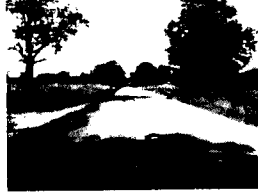
RURAL AREA RESURFACING (SURFACE TREATMENT) PICKERING / UXBRIDGE TOWNLINE
